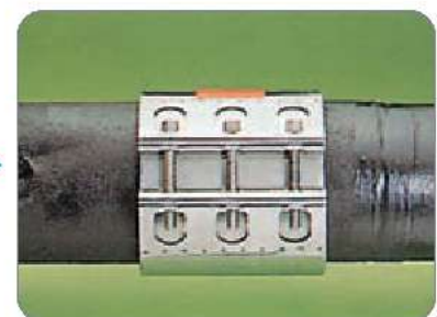
▲COMPLETED THE REPAIRING
