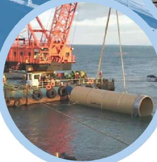
Installation of ocean bed blocks
