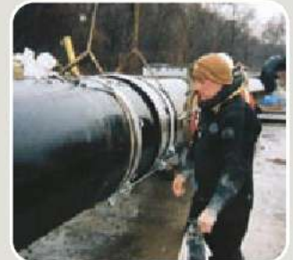
▲ UK: district heating work
