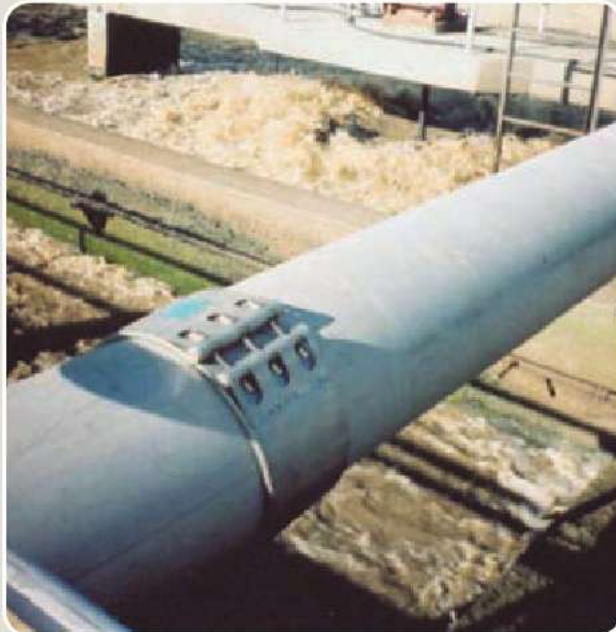
▲ Spain: water purification facilities
