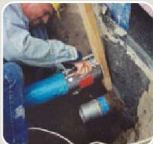
▲ U.S.: sewerage repair work
