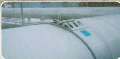
▲ 48" (1,200A) MF-RL Canadian power plant cooling line
