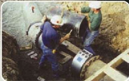
▲ Repair work for pipes replaced underground
