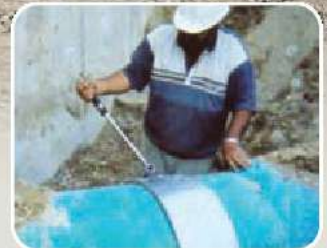
▲ UK: buried water supply pipes
