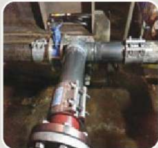
▲ Netherland desalination treatment facilities
