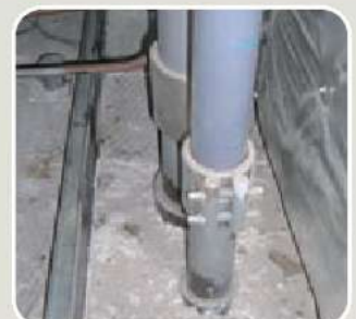
▲ PVC + Steel Pipe Connection
