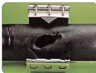
▲REPAIRING THE PIPES
