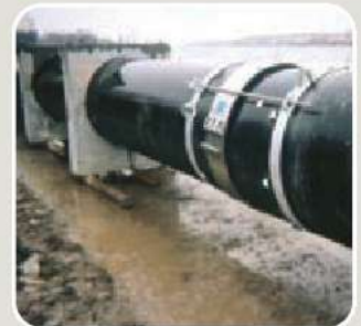
▲ U.S.: nuclear power plant
