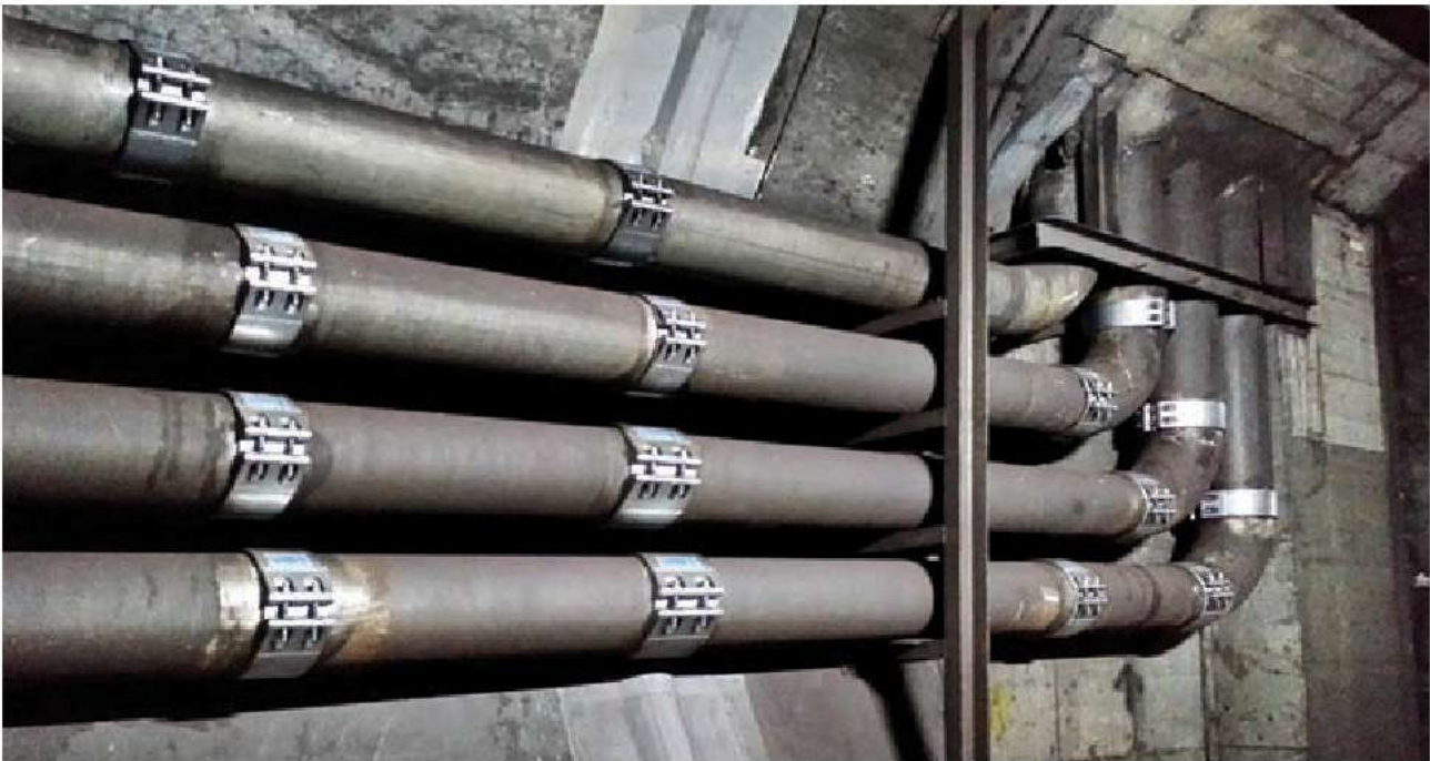
▲ Underground drainage repair(Maintenance) works
